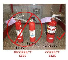
The correct size, 2A:10BC, is larger than the 10BC and 1A:10BC fire extinguishers and it typically has a flexible hose and nozzle which requires 2 hands to operate. You can operate the fire extinguisher by remembering the acronym PASS-Pull, Aim, Squeeze and Sweep. To watch a video on how to operate a fire extinguisher, click here: <a href="https://youtu.be/GVBamXXVD30?si=jy3ryU4Ii-WAmLVC">https://youtu.be/GVBamXXVD30?si=jy3ryU4Ii-WAmLVC</a>
